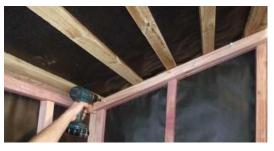
Step 15: Using 2 x 75mm framing nails, nail centre rafter to front and back top plate stiffeners. Predrill if necessary.
