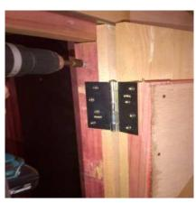
Step 22: Screw padbolt as shown, to the edge of the trailing door, (Left hand door) ensuring padbolt will protrude at least 10mm into Bottom plate in locked position.
