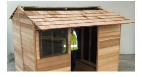
Step 14: Using 75mm tek screws, screw roof panels into end wall panels, (2 screws each end per panel), ensuring end of rafter lines up with centre of gable panel.
